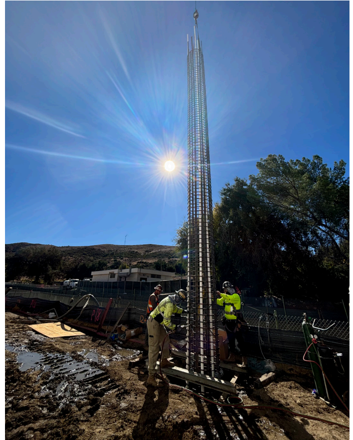
Reinforcement Placement for CIDH Pile.
